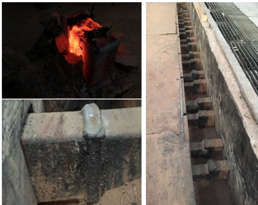
Figure 12. Industrial application of cathode steel collector bar narrow-gap full-section welding.
